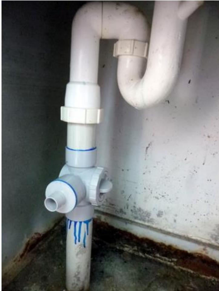
Valve to run laundry effluent to constructed wetland or waste
