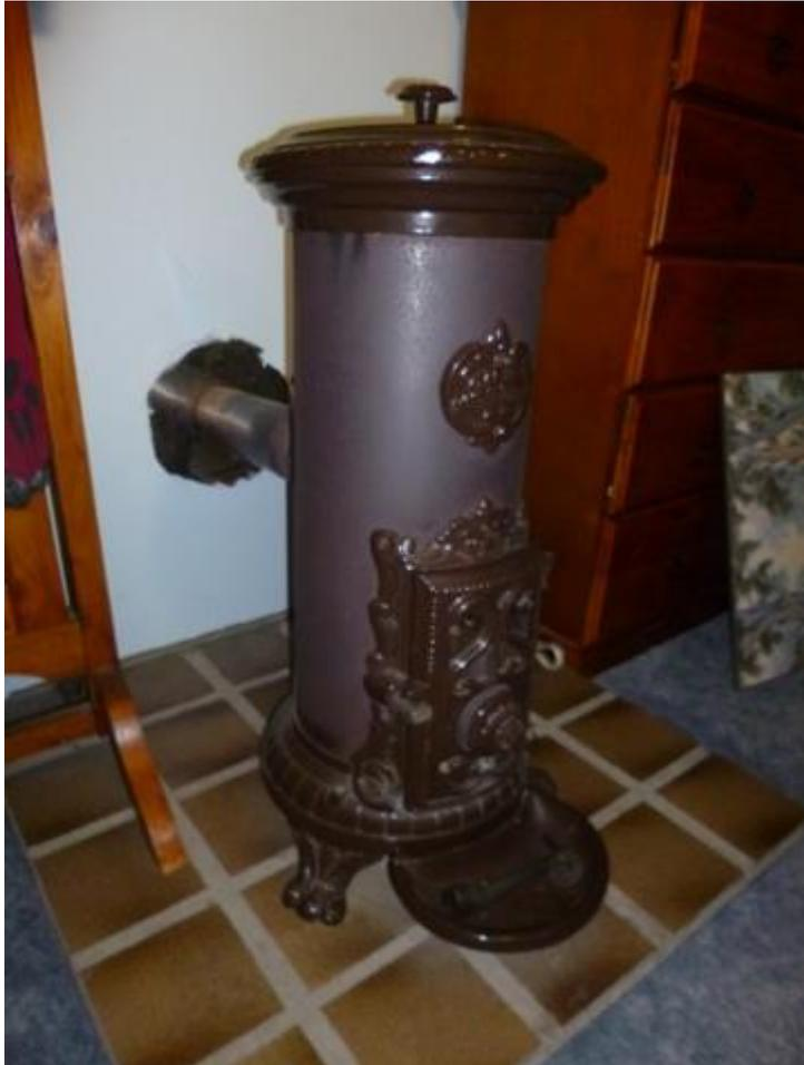
The Godin is a firebrick lined slow combustion heater which could theoretically be used for cooking on the cast iron lid where the wood went in but we never found it to be all that successful, it took forever even to boil water. The Godin is multi-fuel in that you can use wood or coal but we have only used it as a wood stove.
