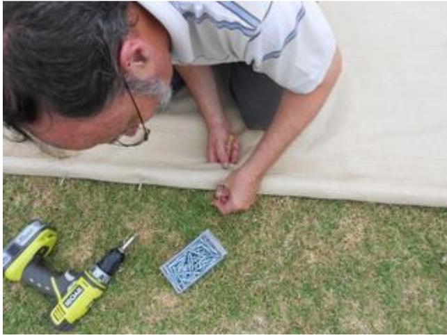
*Using the Bradawl to locate the screw*
