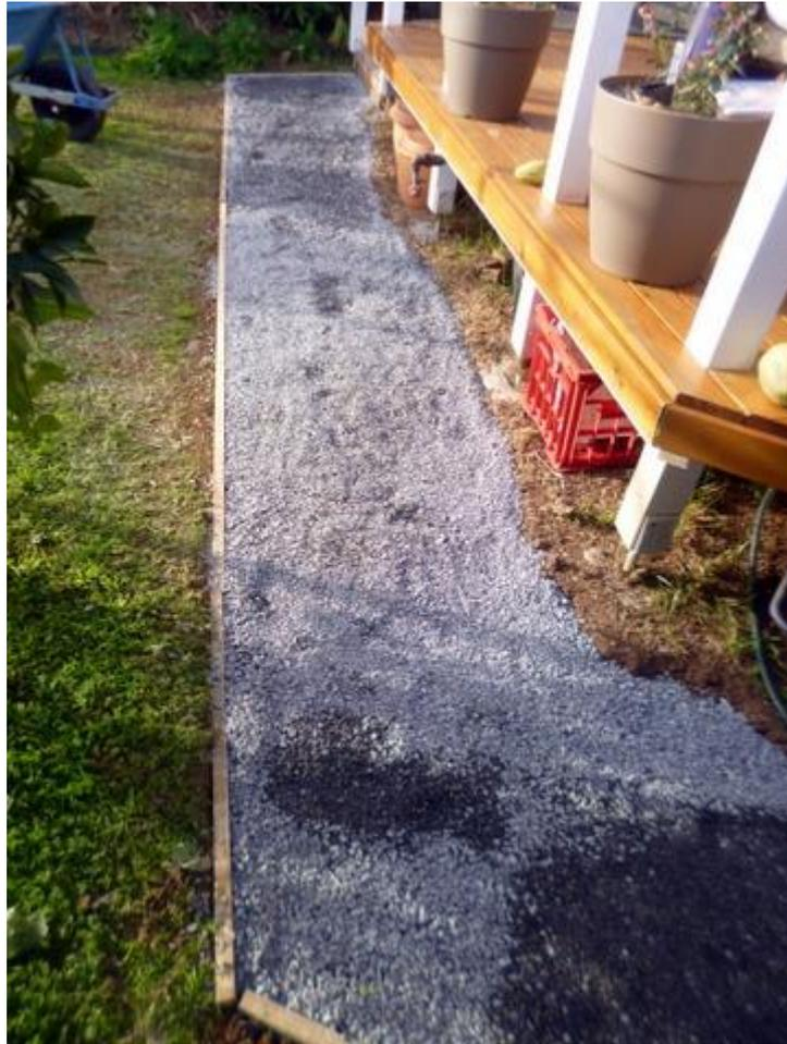
*Our permeable path, taking water from the back deck*
