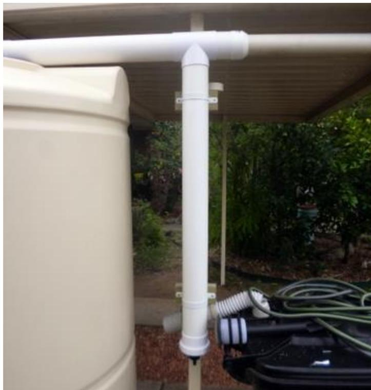
The kit came with a number of orifice plates for the exit of the diverter, with two different size holes, which regulate the speed at which the water drains to re-set the diverter. I picked the smaller of the two types of orifice plates so we will see how that goes.
