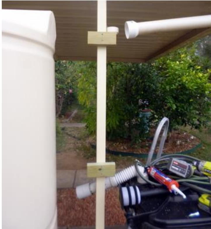
In the event, I could not screw the clips in tight enough and when the diverter filled with rain it was too heavy and started to slip through the clips. To prevent this happening I screwed a piece of timber to the post underneath the end of the vertical pipe such that the edge of the pipe sat on it. This now supports the vertical section and it cannot move down due to gravity.
