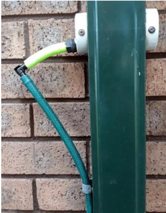
After the above was written I did tweak it a bit. Rather than having the hose stick straight out I inserted a corner piece and screwed the hose to the downpipe with a couple of conduit half saddles to secure it. I then ran the hose long the back wall of the house and under the wood chip and bark to conceal it, just poking the end out over the bathtub. I checked and it worked!
