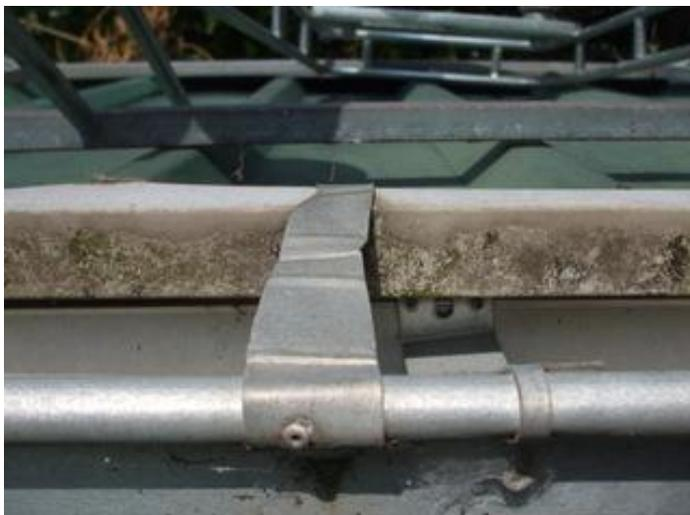
This shot shows a brace, pop riveted on the roof, curled around the gutter and pop riveted to the gutter
