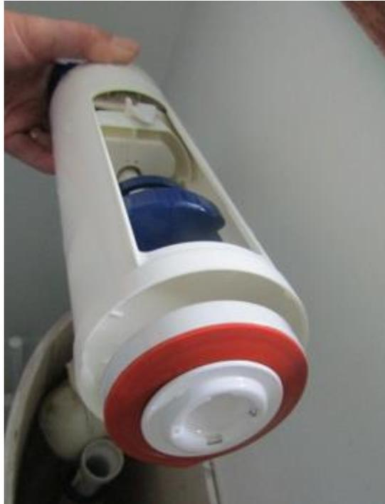
*The orange flush valve washer at the base of the dual flush mechanism*
