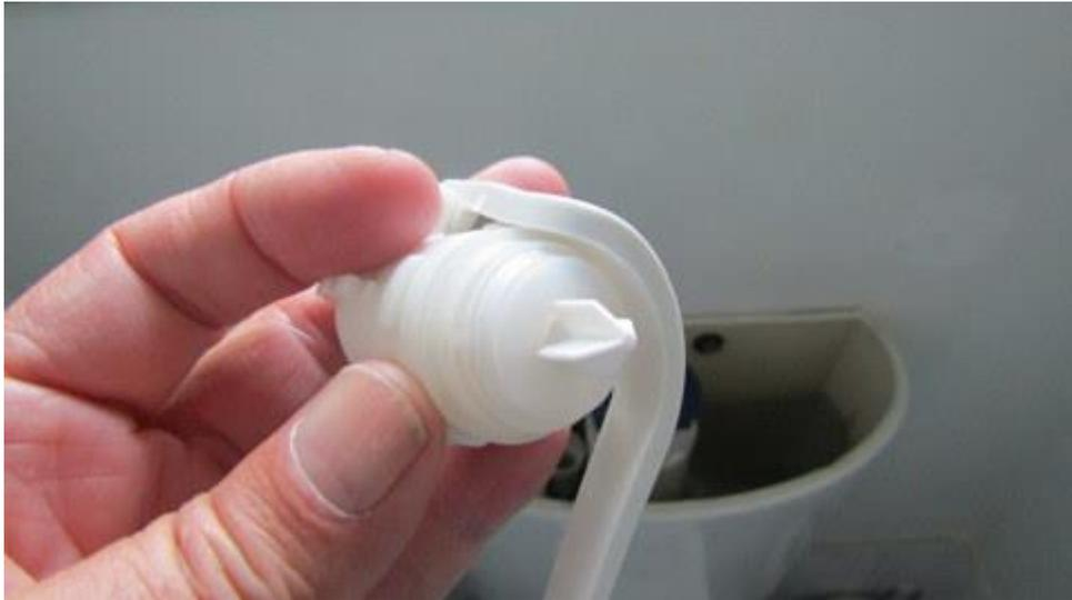
*New inlet valve headseal in place and about to be refitted into the cistern*
