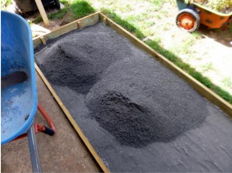
With the surround in place I worked out the volume (0.8m<sup>3</sup>) and after discussion with a supplier, bought in 1.5 tonnes of blue metal dust (also referred to by some as just “metal dust”). I barrowed in the metal dust in layers, using my weight to compact the blue metal dust between layers (ie after each layer I stomped it down – crude, but effective). I then smoothed off the top level with the timber surround, which I had previously levelled with a spirit level.
