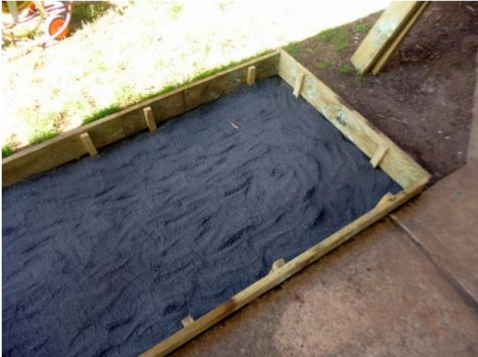
With the hole dug so that it was 50mm bigger than the tank footprint all around, I lined the edges with some 150mm wide x 28mm thick x 4000mm long CCA boards. Due to the slope of the land the eastern end was practically buried while the western end was about 100mm above the ground. I got hold of some 400mm stakes and placed the boards where they were supposed to go, drove in the stakes behind them, then screwed the stakes to the boards with 50mm screws. This gave me a good, solid surround.
