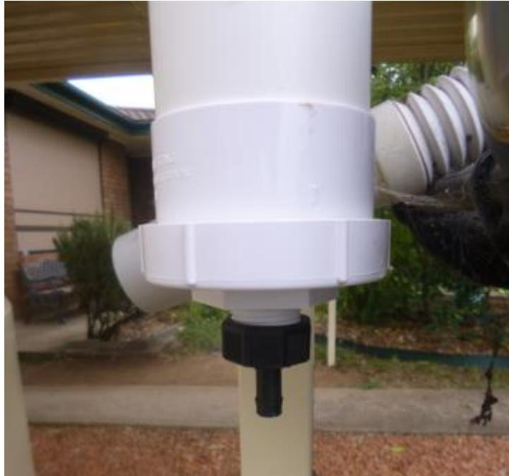
I assembled the diverter without using any glue (so that if I screwed it up I could pull it apart and re-do it) but it seems to be working well, all we need now is some rain to fill the tank! Due to the lack of rain for the past few months I have not put in an overflow on the tank just yet, the tank has barely a few centimetres of rain in the bottom so far, just enough to reach the bottom tap.
