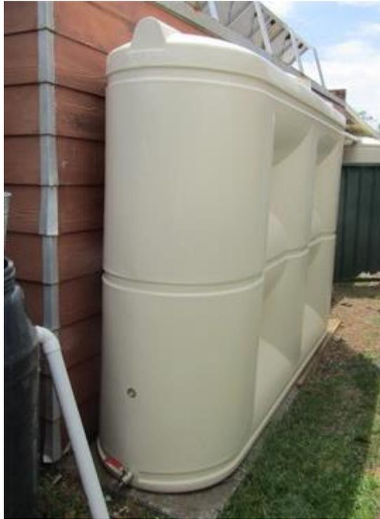
The only things left to do were to drill out and fit the valve in the bottom of the tank and install the overflow to the 3000 litre tank, which I did.
