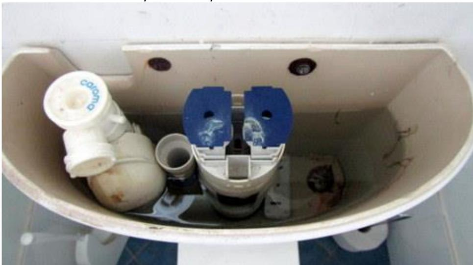
*The view inside our cistern - white structure on the left is the inlet, open tube in the middles is the internal overflow and the cylinder on the right is the dual flush mechanism.*
