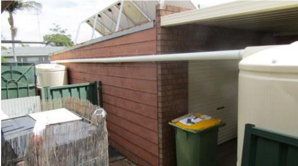
The inlet of the new tank was in the centre of the top of the tank and about 7 metres away from the 5000litre tank. I used 90mm stormwater piping running from the outlet of the first tank to the inlet of the new one. I didn't have a 90mm hole saw to drill the outlet hole in the 5000 litre tank but I did have a 65mm one and figured that would do the trick (which in fact it did!).
