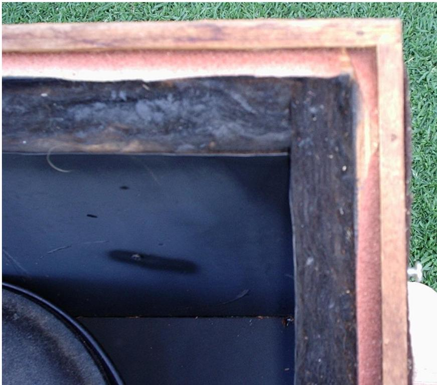
*Detail of corner showing steel, insulation, felt and timber*
