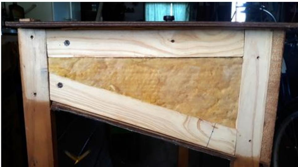
*The side with cover removed showing insulation in place*
