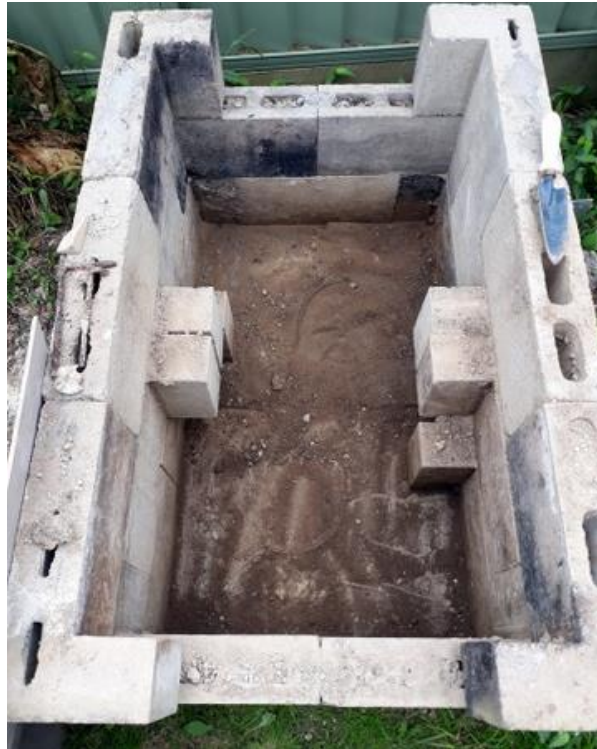
Empty and ready for demo!
