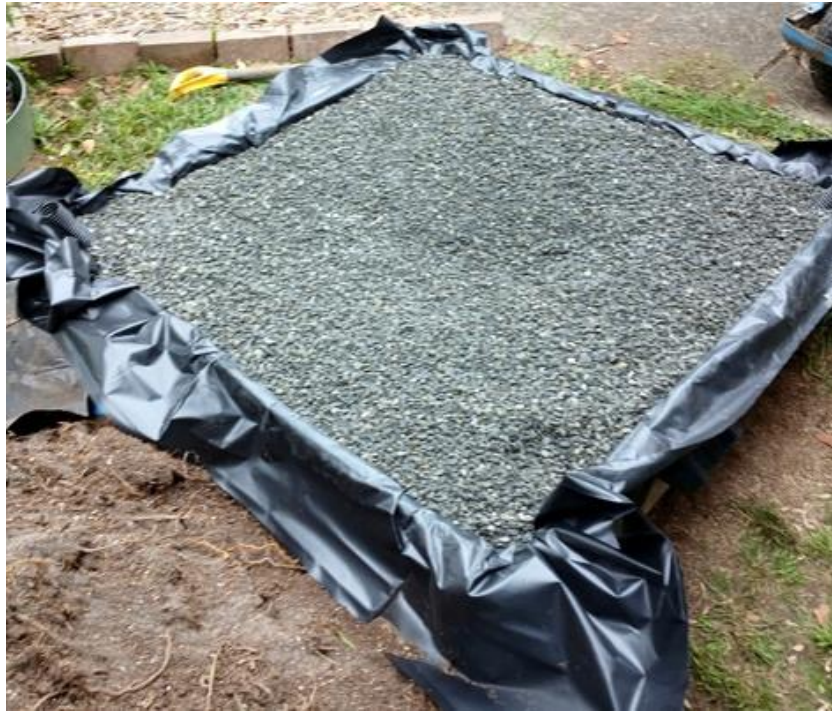
New plastic membrane, 10mm gravel and ag pipe watering point installed
