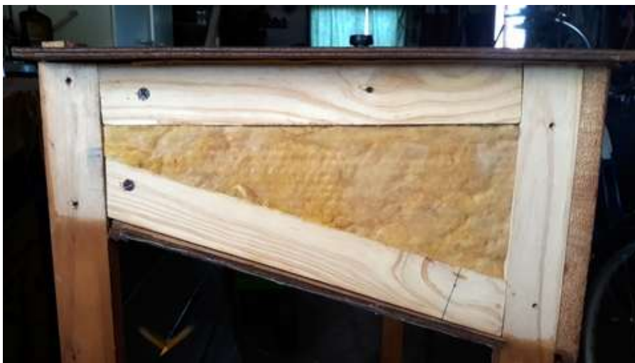
The side with cover removed showing insulation in place
