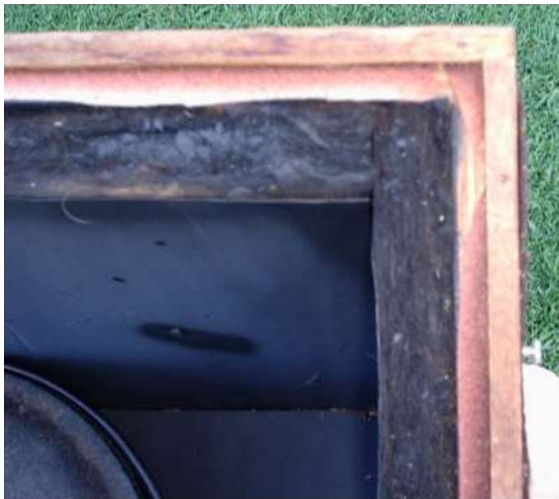
Detail of corner showing steel, insulation, felt and timber
