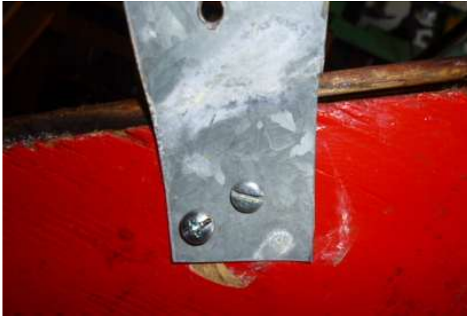
Installing the second screw to stop the attachment from rotating
